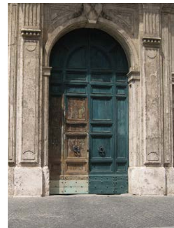
Portone Prima del restauro Main entrance door before restoration.
