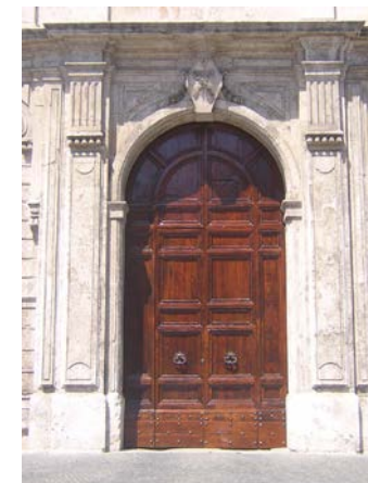
Portone dopo del restauro, 2008. Main entrance door after resto- ration, 2008.
